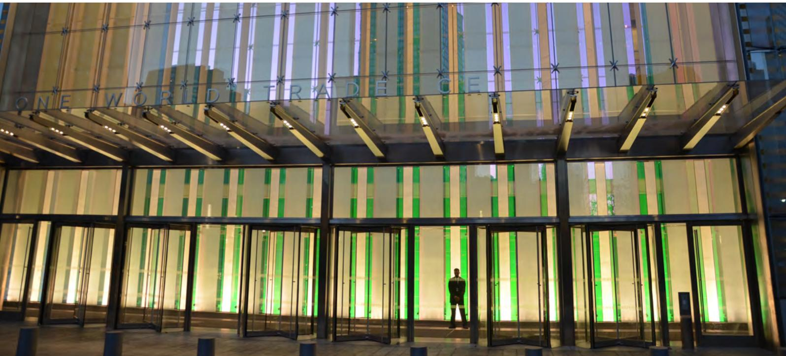
dichroic filters are let into the long sides of the panes as a 20 cm wide strip, which allows intense green light into the building and reflects violet light.
